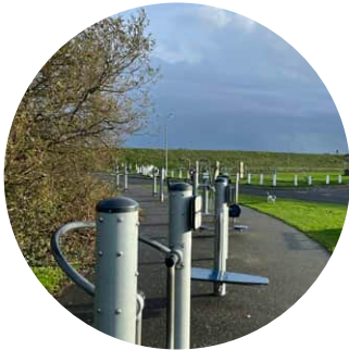
OUTDOOR GYM EQUIPMENT Refurbished and consolidated on site
